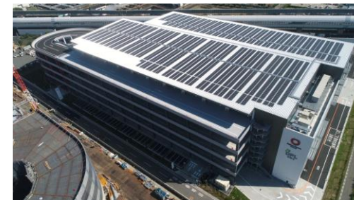
Rooftop solar panel (logistics facilities)
