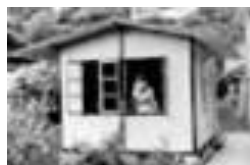
1959 Midget House As a study room which could be constructed in three hours helped the solution to housing space shortage caused by rising birthrate
