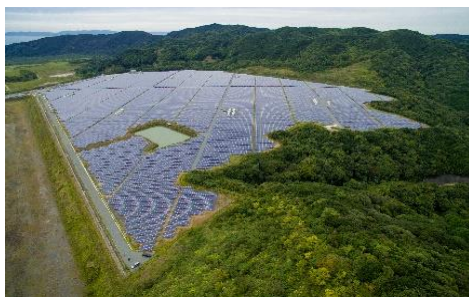
Solar power generation
